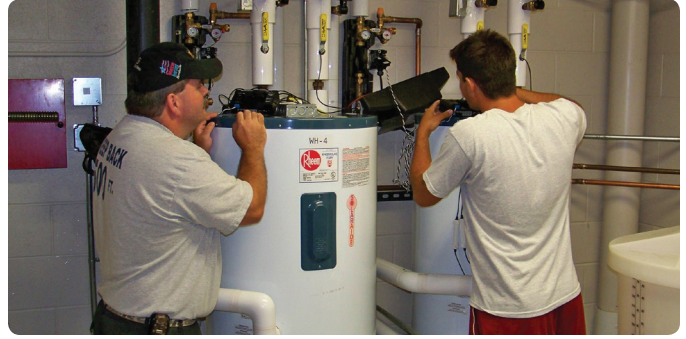
St. Clair County Community College students use data loggers to measure and analyze water temperatures as part of the new Siemens solar-powered hot water system in the college's Acheson Technology Center.
