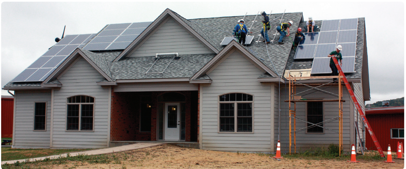
Students help to install solar panels atop Alfred State's net-zero model home.
