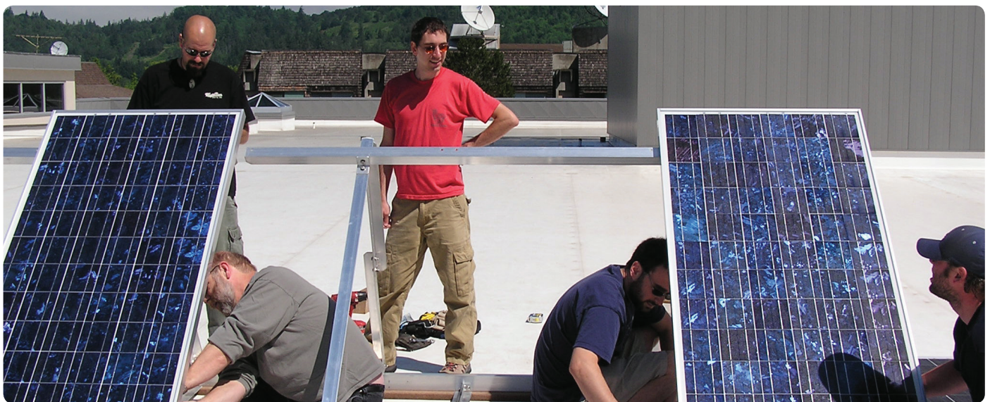
Students install a 1 kW solar PV system on the Lane Community College science building roof.
