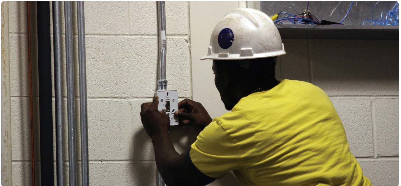
A building automation student mounts a sensor in GPTC's Green Technologies Academy.
