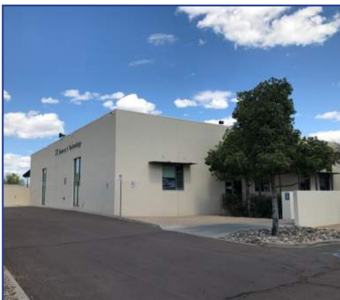
Existing Auto Lab - Exterior
